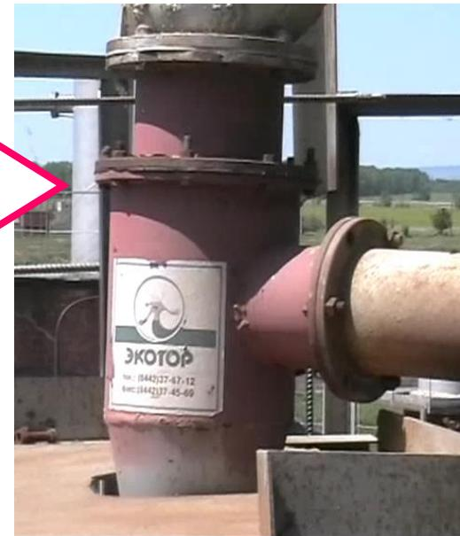
A pipeline installation providing uniform mixing of the sludge, is mounted inside the digesters
