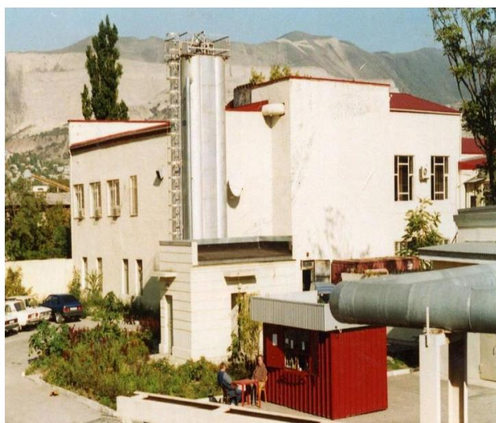
City WWTP 4000 m<sup>3</sup>/day, Tashkent region, Uzbekistan. Sludge treatment – by a separate reactor
